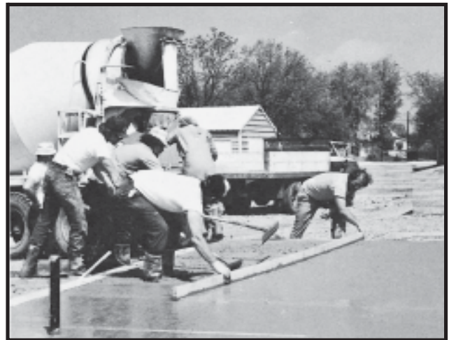
Finishing Concrete Flatwork
